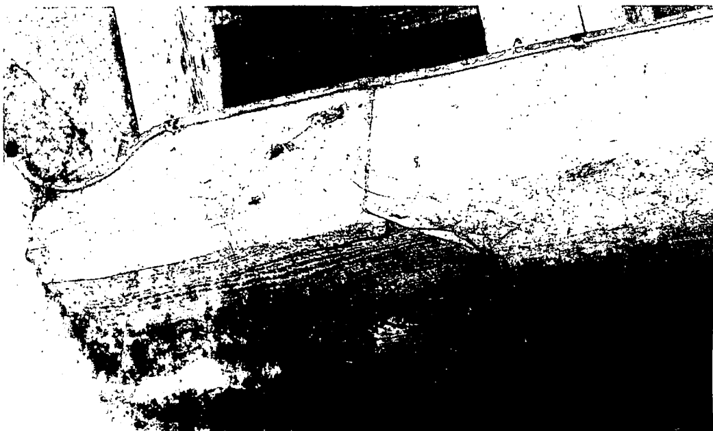
Fig 34. Type 2 scarf joint in wall-plate.
