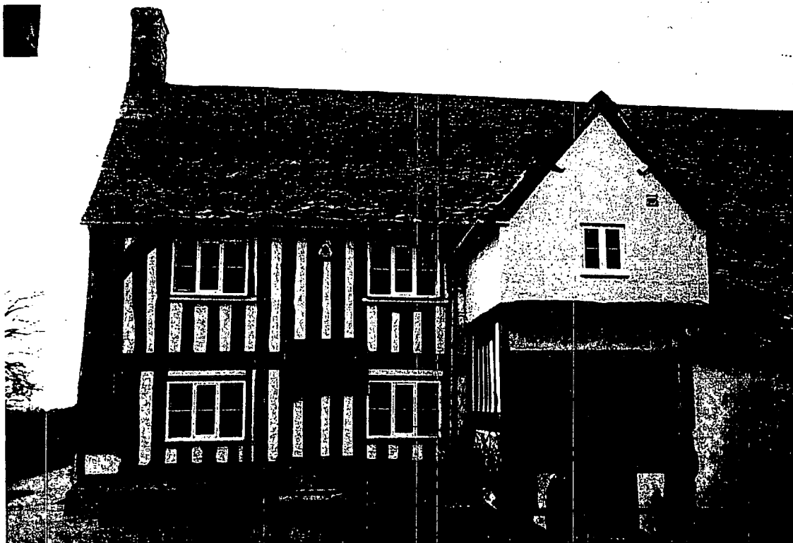
Fig 3. Church Farm, South Leigh. House from north. Note close studding, two storied porch and stone plinth.
